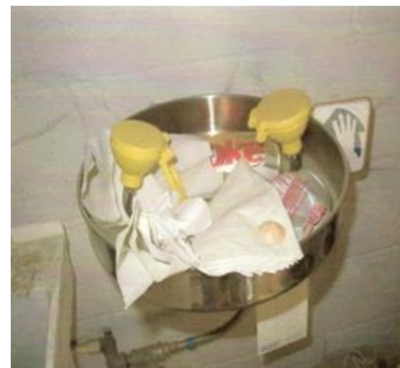
Example of an eyewash station that was not kept clear of debris nor tested weekly.
